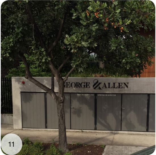
Fire hydrant services box with ground covers in front & shrubs behind
